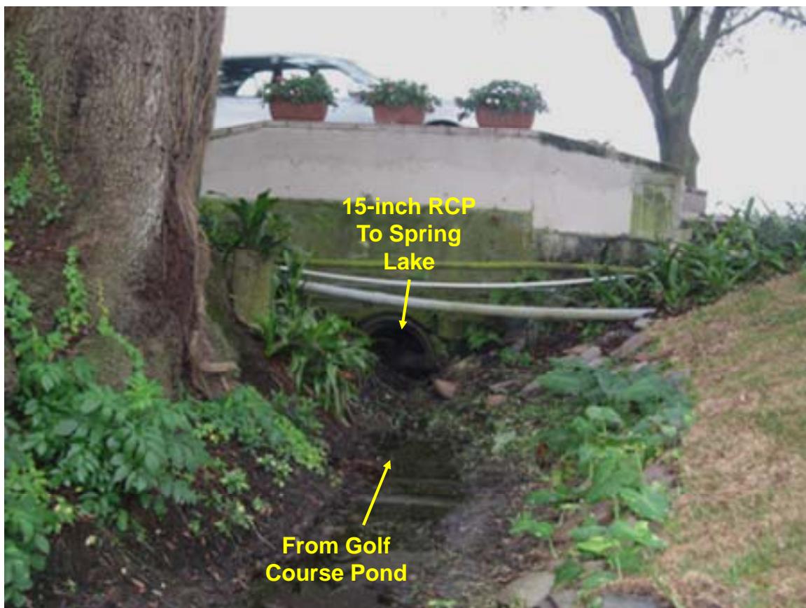
Figure 5-10b. Photograph of Earthen Ditch Terminating into a 15-inch RCP.
