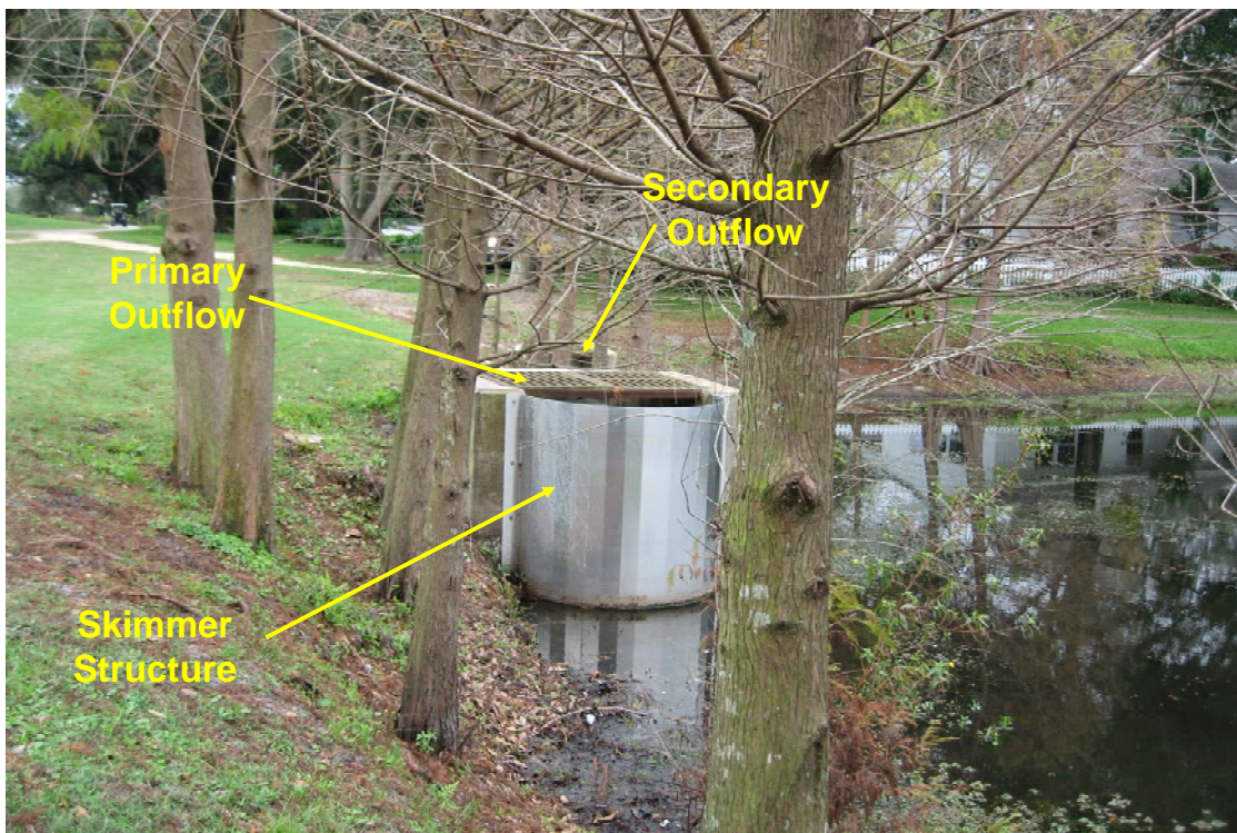
Figure 5-7. Photograph of the Two Outfall Structures at Site 3.
