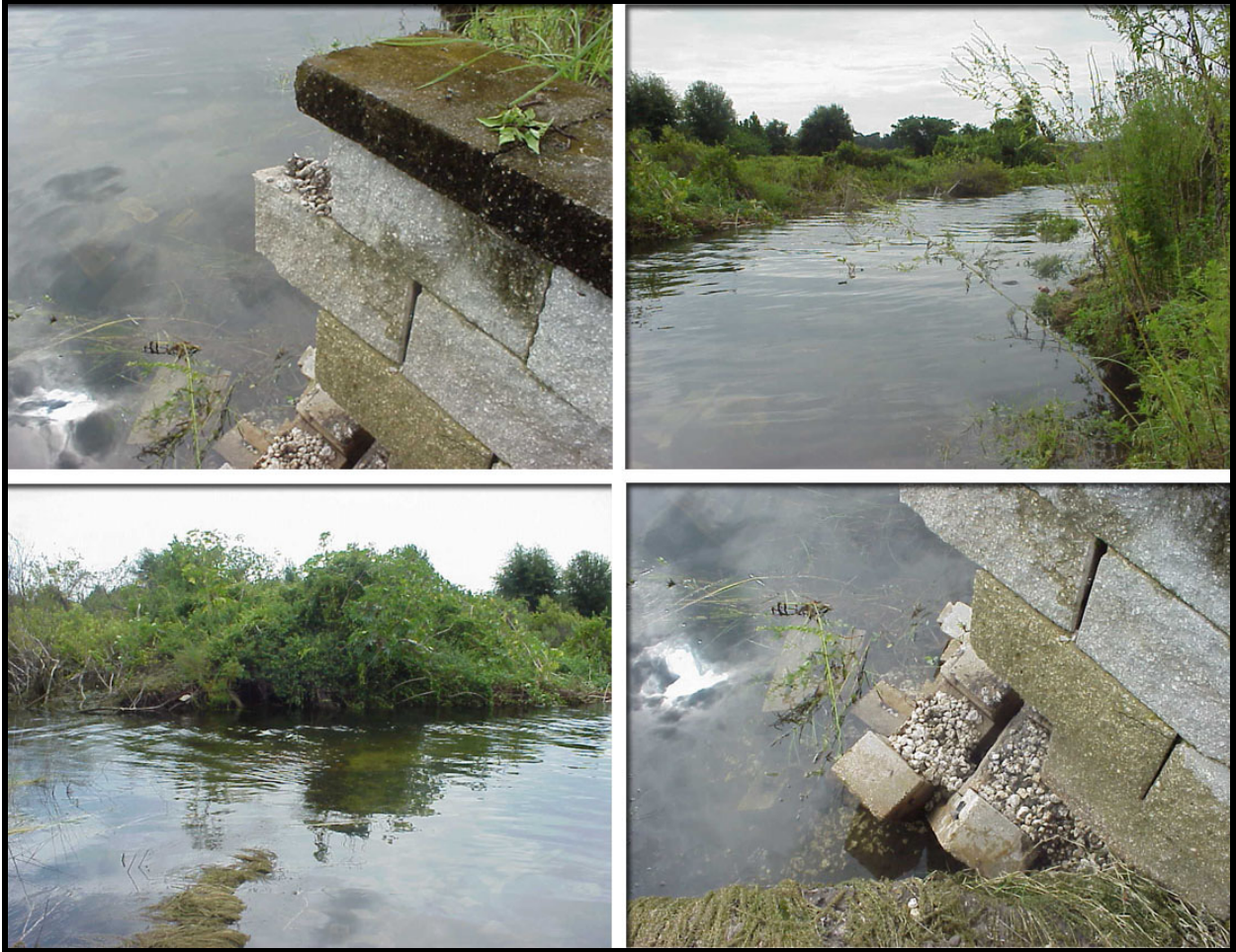
Photo 3. Vizcaya Condo Retaining Wall Failure (August 2003; courtesy Orange County)
