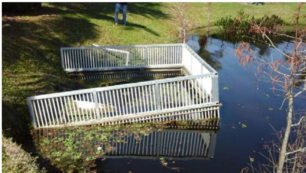
Figure 2-34. Outfall Structure for Lake Roberts with fish gates
