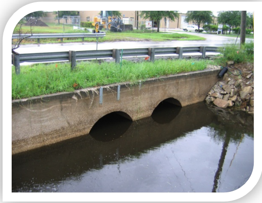
Before – Existing double 77in x 52in culverts at Central Florida Parkway.
