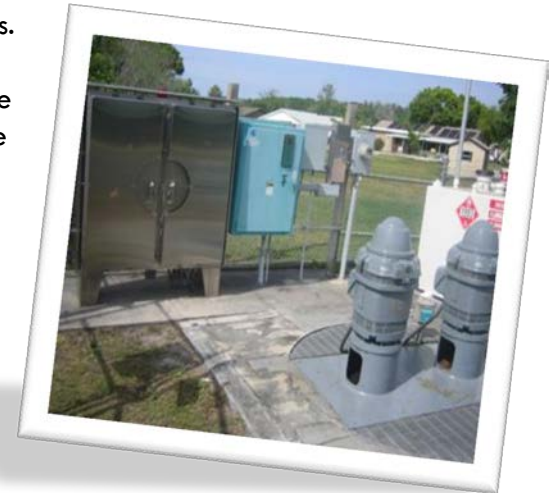
PUMP STATION MOTORS
