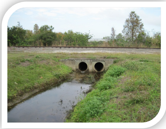
Before - Existing 48in steel culverts at railroad crossing.
