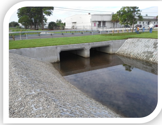
After – Double 10ft x 5ft concrete box culverts.
