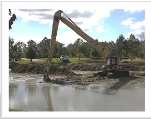
BANK REGRADE AND REPAIR
