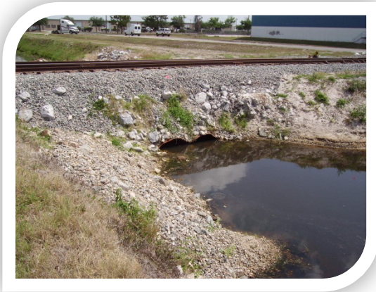
Before – Existing double 48in culverts at southern railroad spur.
