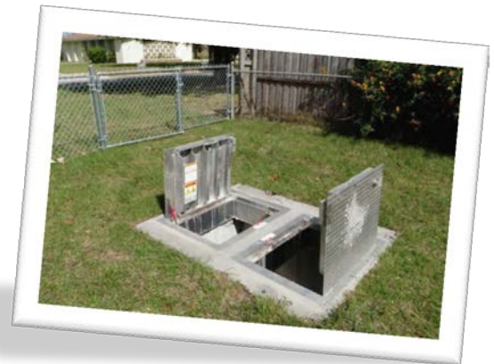
DRAINWELL ACCESS VAULT
