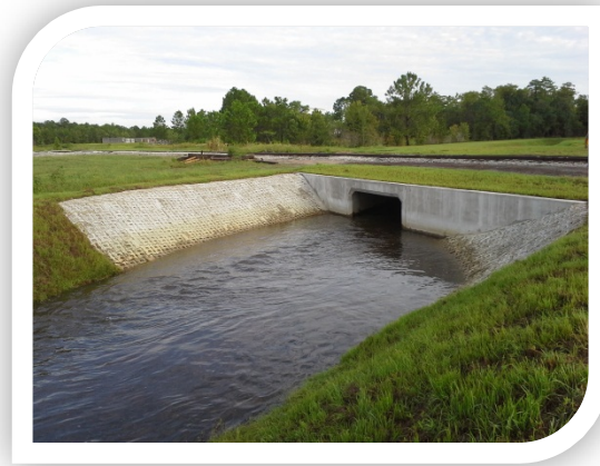
After – Large 10ft x 5ft concrete box culvert installed.
