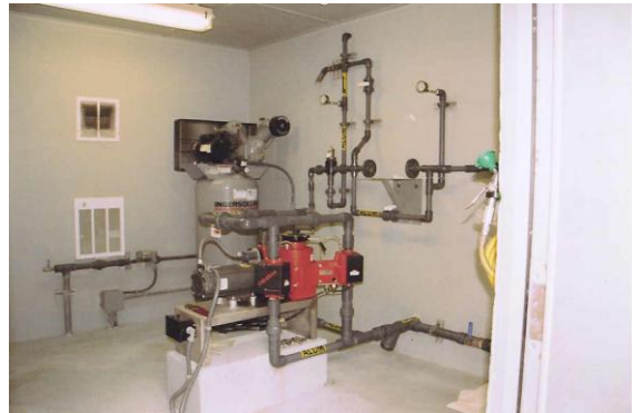
Mead Garden alum injection station
