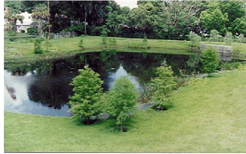
Traditional wet retention/detention pond
